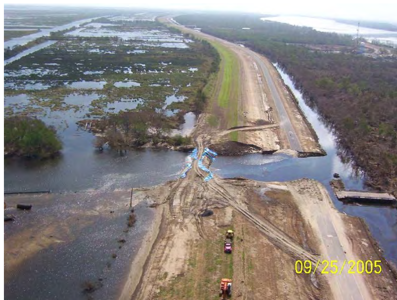
Figure 5.4: Aerial photograph of levee breach of hurricane (back) levee east of Pointe a la Hache (September 25, 2005)
