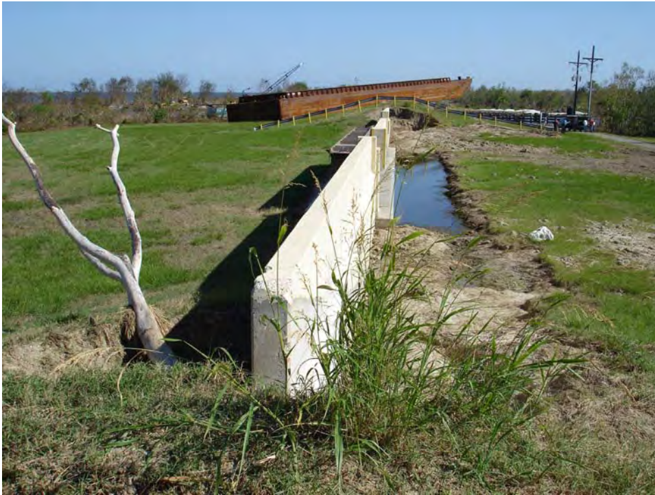
Fig. 4.15, Scour near Bienvenue Gate site (L. Wooten, October 5, 2005).
