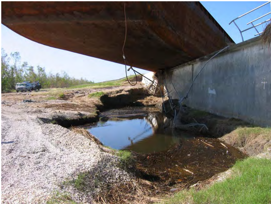
Fig. 4.14: Scour near barge damage at the Bienvenue Gate site (J. Wartman, October 5, 2005).
