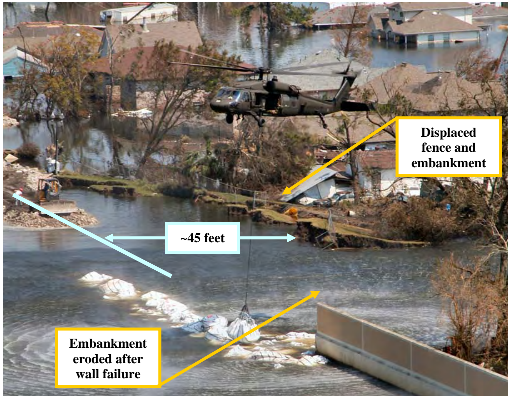
Figure 2.3(b): The 17 th Street breach, highlighting key points for discussion
