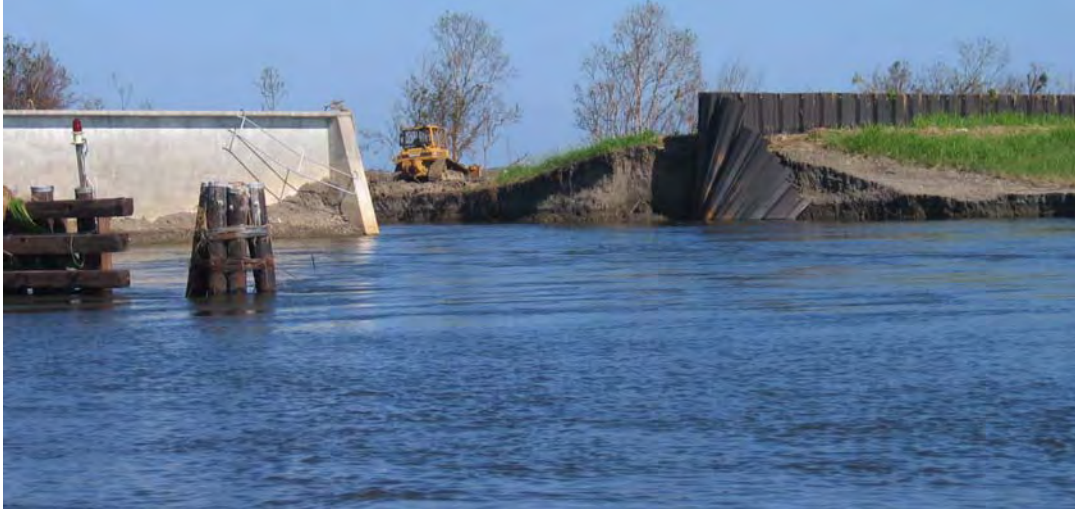
Fig. 4.13: Sheet pile breach at the Bayou Bienvenue Gate (J. Wartman, October 5, 2005).
