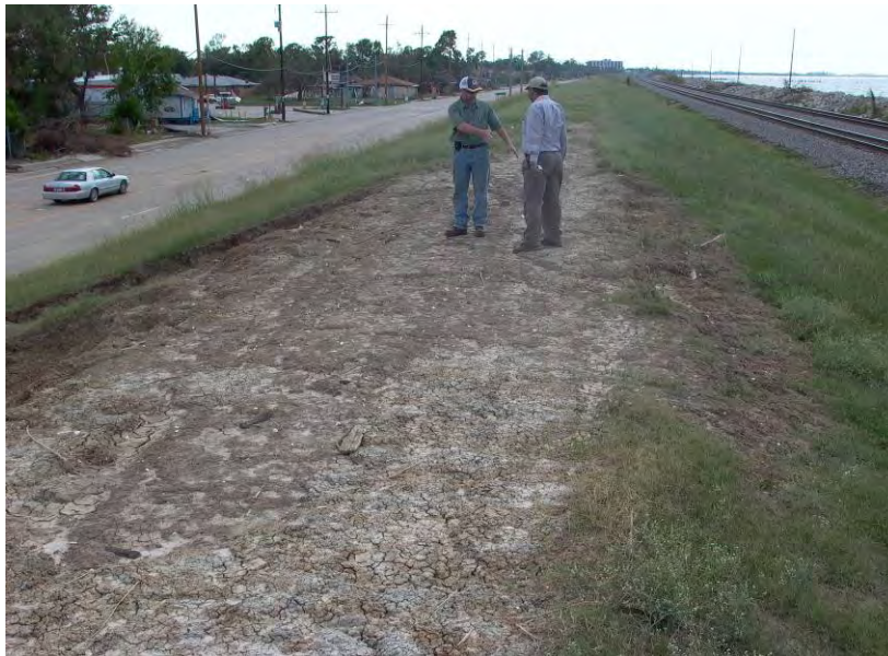
Figure 3.6: Wave overtopping of lakefront earthen levee at low spot in structure did not cause serious damage (Photo by F. Silva – N 30° 03' 47.8", W 89° 58' 13.1)
