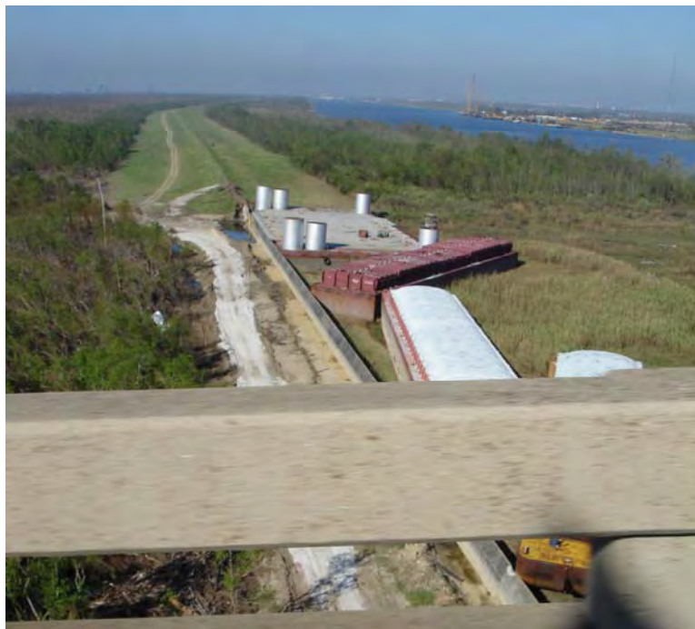
Fig. 4.16, View of levee along the south bank of the Intracoastal Waterway from the Rt. 47 Bridge. (Lee Wooten, October 6, 2005)
