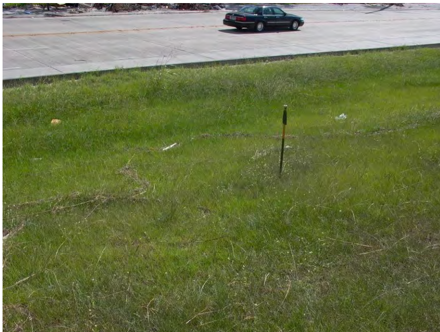
Figure 3.7: Debris line indicating prior sheet flow, most likely from wave overtopping or “splash-over”, on landside slope of lakefront levee (Photo by F. Silva – N 30° 03' 47.8". W 89° 58' 13.1")
