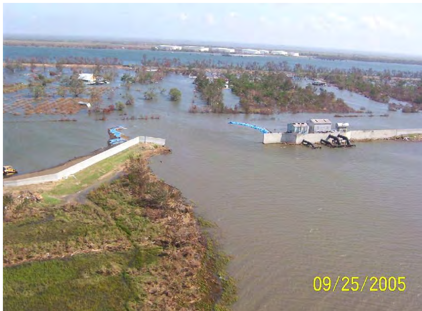
Figure 5.2: Aerial photograph of levee breach of hurricane (back) levee along western side of the Mississippi River near the community of Sunrise (September 25, 2005)
