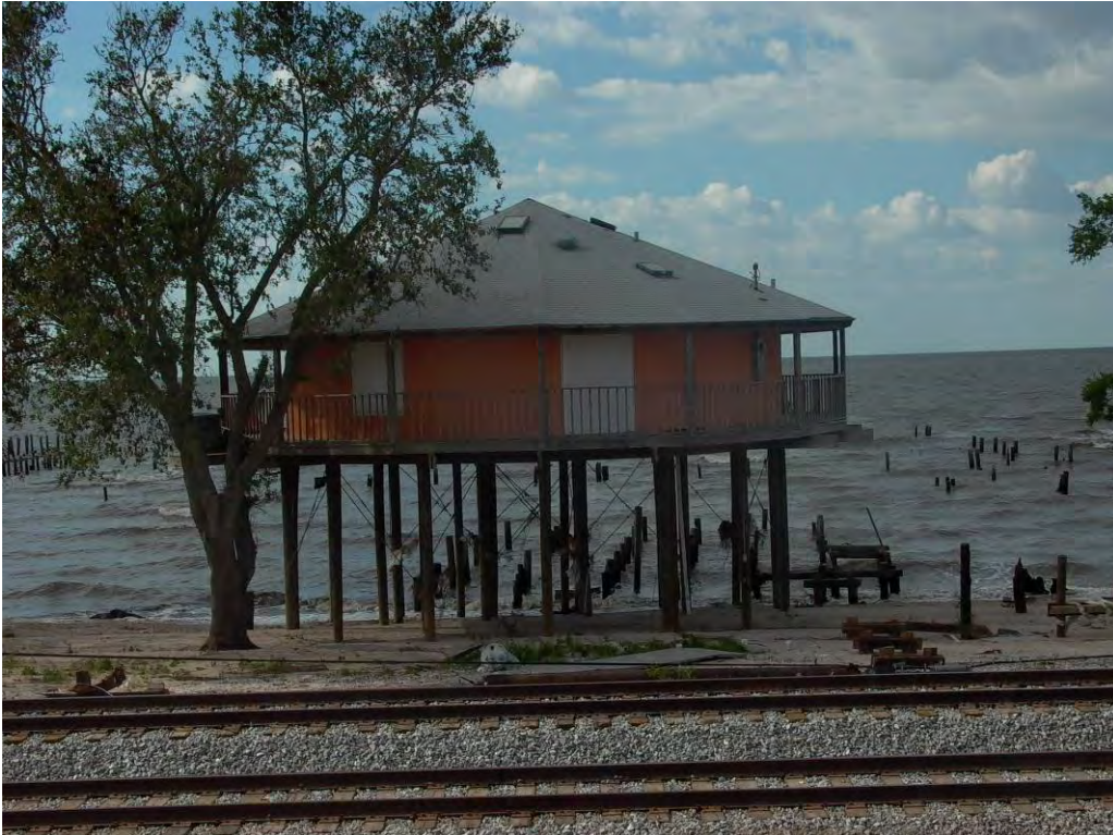
Figure 3.10: The lone surviving structure at Little Woods appears unscathed, except for the lack of stairs. (Photo by F. Silva)
