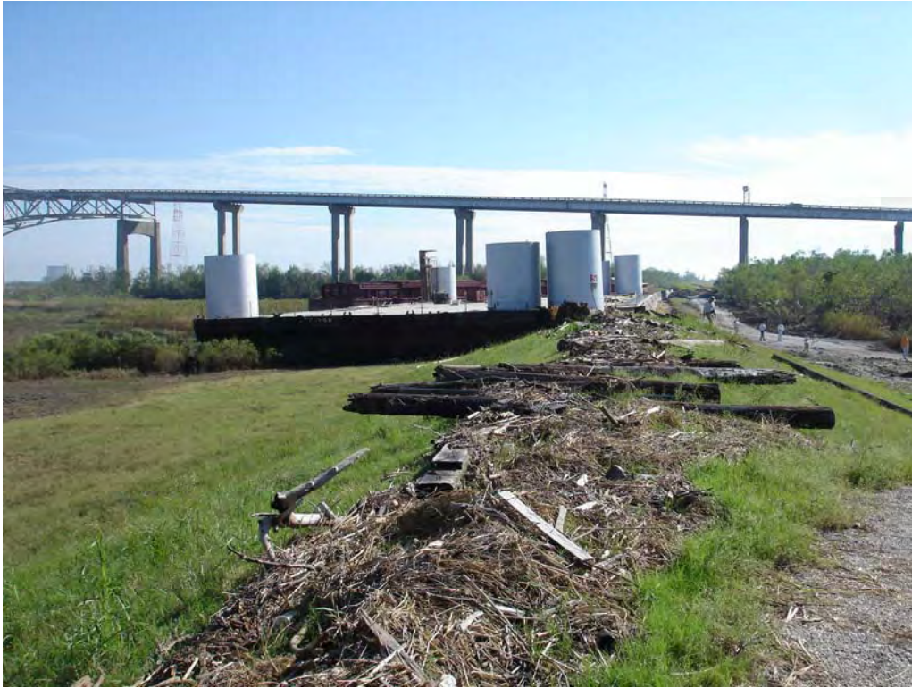
Fig. 17: Debris line near levee crest just west of the Rt. 47 Bridge south abutment. (L. Wooten, October 5, 2005).
