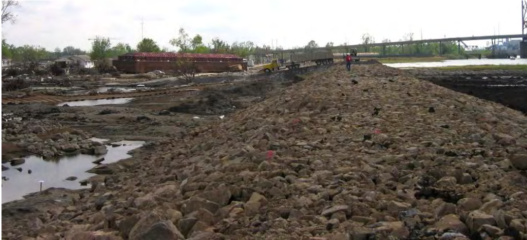
Fig. 4.6 - South view of the south breach repair at the Lower Ninth Ward (J. Wartman, October 4, 2005).
