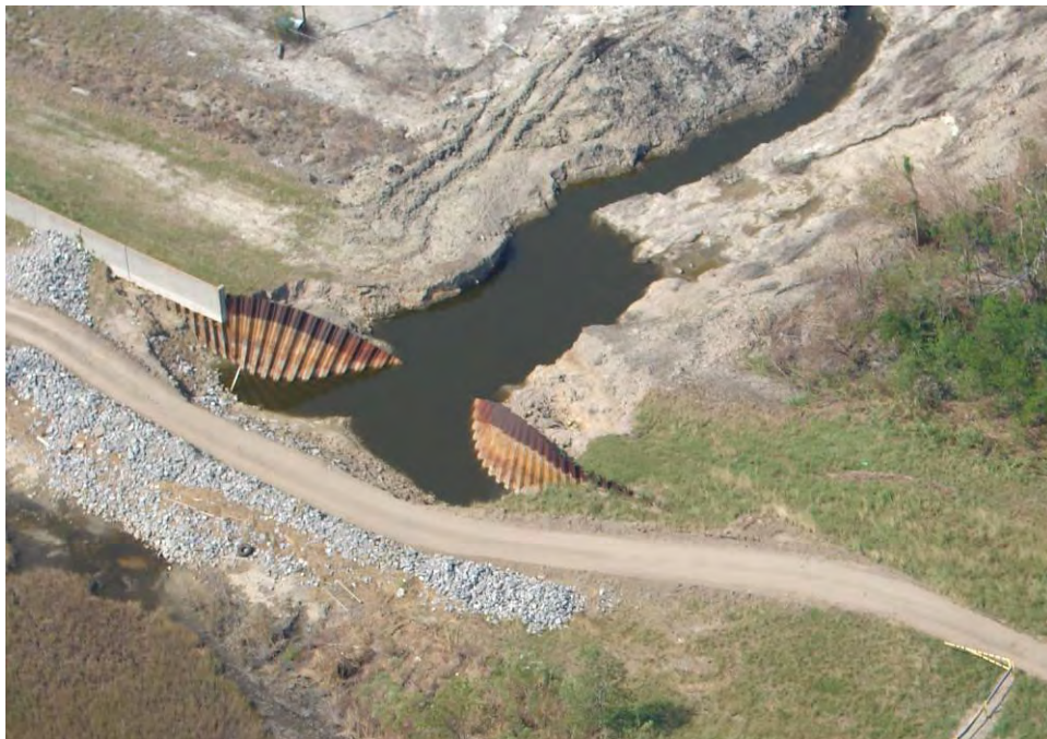
Figure 3.14: Aerial view of the failed wall section shown in Figure 3.13
