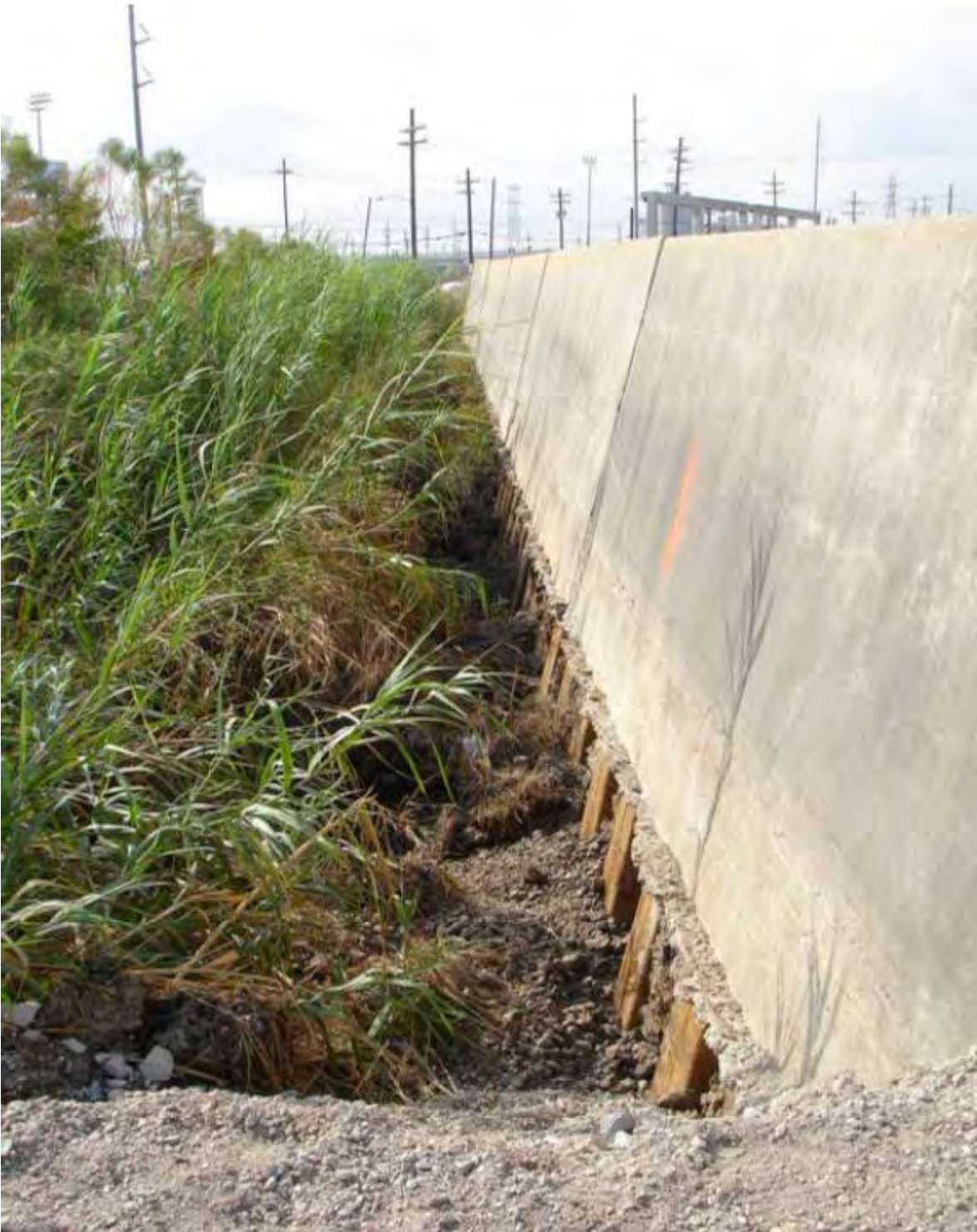
Figure 3.12: “Gapping” between soil and wall as distressed wall was displaced landward from the Intracoastal Waterway.
