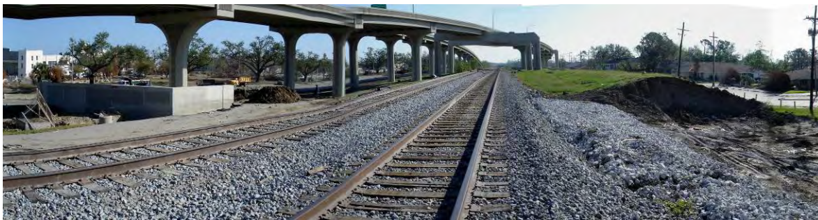
Figure 3.2: Complex transition near Lakefront Airport consisting of various flood protection heights, differing materials and junctures between various jurisdictional organizations. These types of complex transitions were found to be associated with several of the levee flood protection problems.
