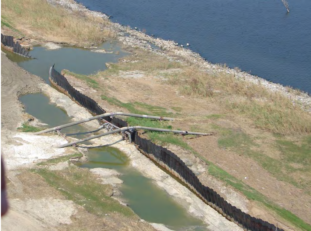
Fig. 21, Levee failure on southwestern bank of MRGO between Bayou Bienvenue (where barge is aground on I-wall) and Bayou Dupree. Note severe erosion and scouring ( L. Harder, October 14, 2005).
