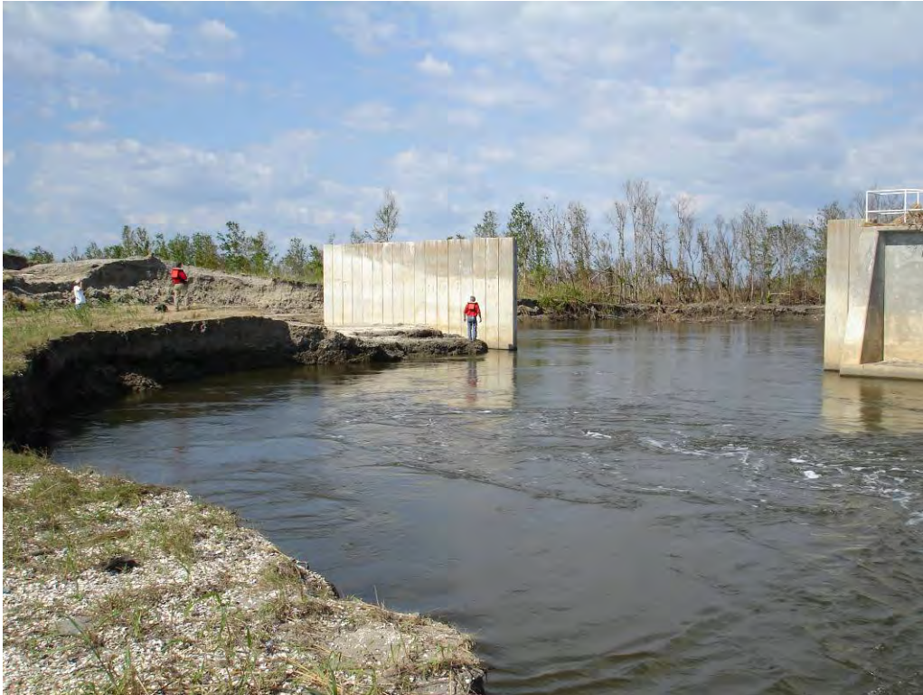
Fig. 23: Ground perspective of Bayou Dupree lock abutment failure (L. Wooten, October 6, 2005).
