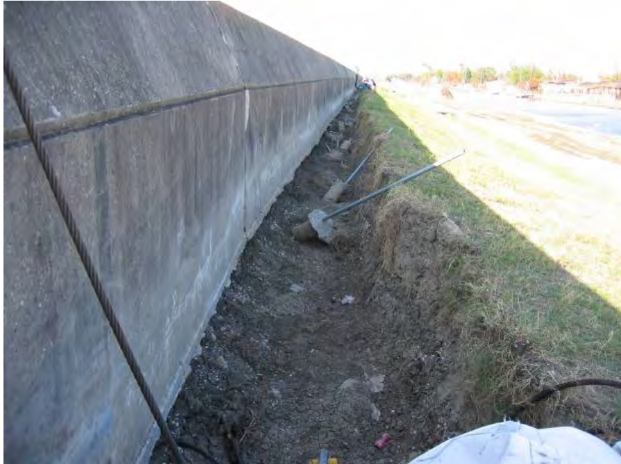
Fig. 4.4: North view from the end of the south breach of Lower Ninth Ward. Note how the scour trench becomes progressively wider as it approaches the breach. (J. Wartman, October 4, 2005).
