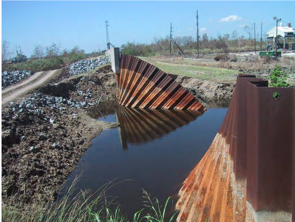
Figure 3.13 Failure of sheetpile wall adjacent to higher and stronger concrete topped I-wall on the north side of the IW.
