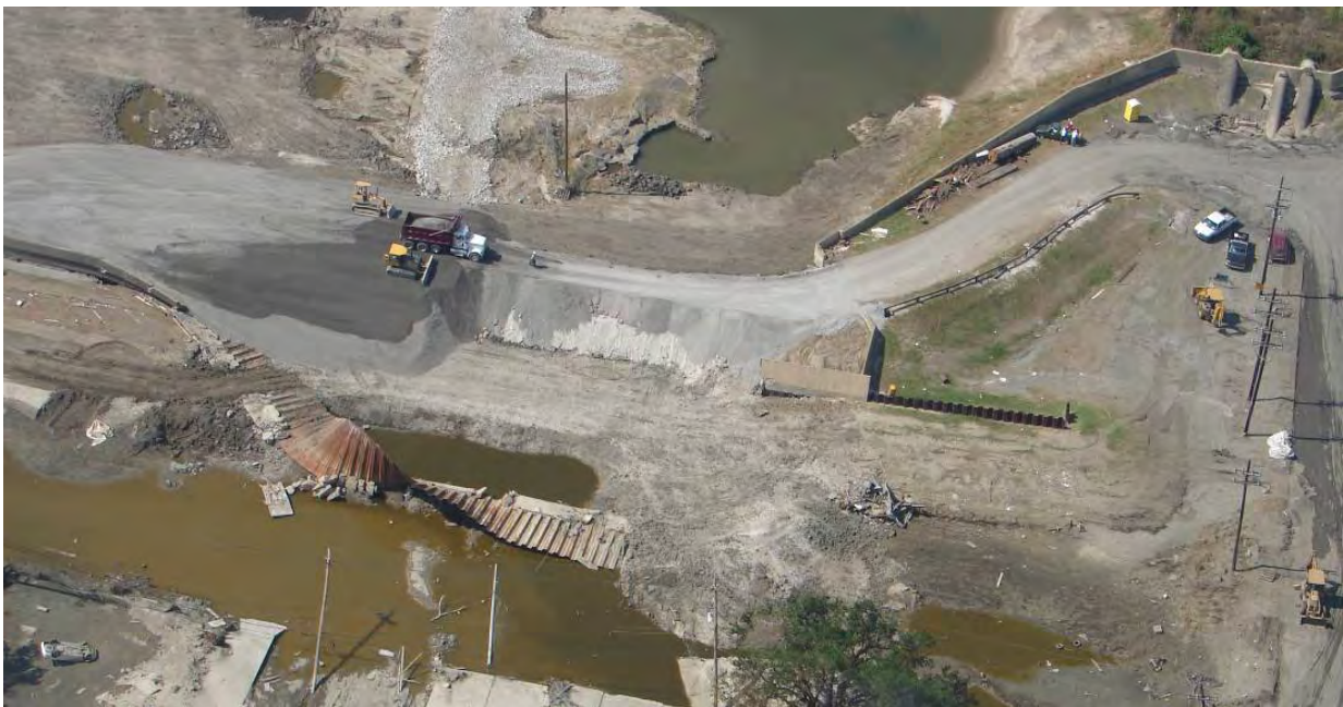
Fig. 4.9: Aerial view of the north breach of the Lower Ninth Ward (L. Harder, October 14, 2005).
