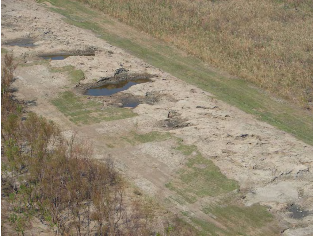
Fig. 25: Overtopping obliterated earth levee along southwestern bank of MRGO, within two miles southeast of Bayou Dupree. Note deep scour at the levee foundation level. (L. Harder, October 14, 2005).
