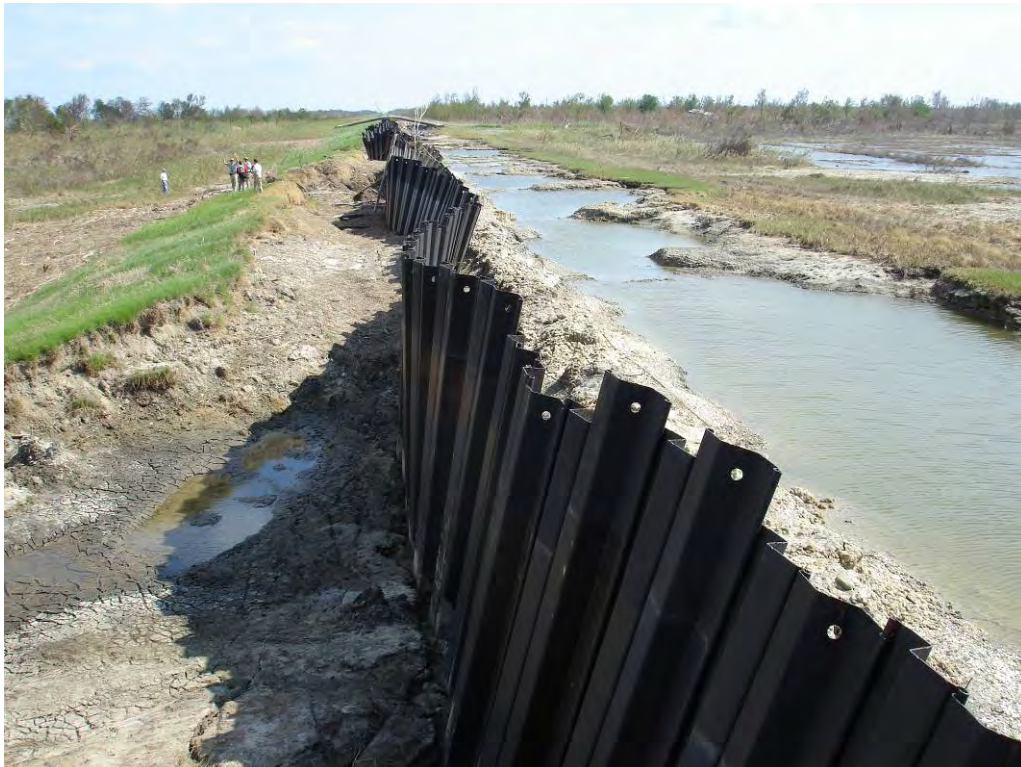
Fig. 20, Failure of earth levee with steel sheetpile barrier on the southeast bank of the MRGO. Note severe erosion and scour (L. Wooten, October 6, 2005).
