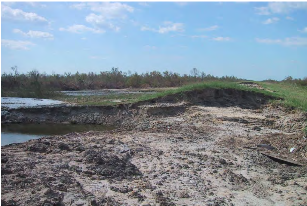
Fig. 24: Failure of earth levee on Southwest bank of MRGO adjacent to the Bayou Dupree gate (L. Wooten, October 6, 2005).
