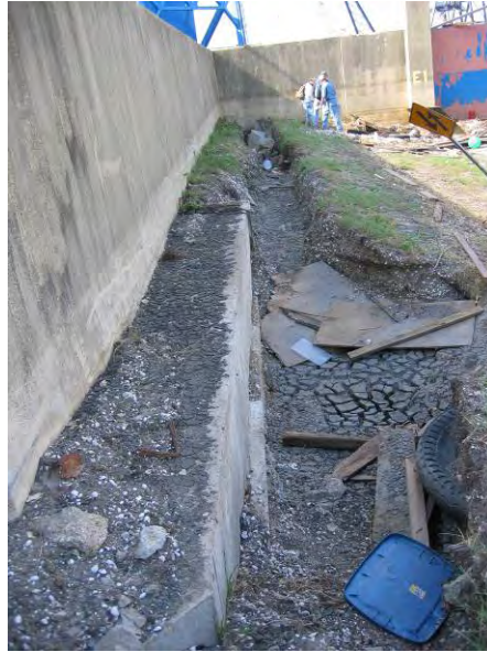
Fig. 4.8 - A scoured, but nevertheless well-performing "T-wall" levee section located near the north breach of the Lower Ninth Ward (J. Wartman, October 4, 2005).
