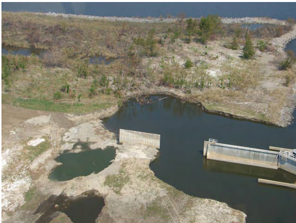
Fig. 22, Levee failure on southwestern bank of MRGO at Bayou Dupree. Note concrete sheetpile and levee transition washouts. (L. Harder, October 14, 2005).
