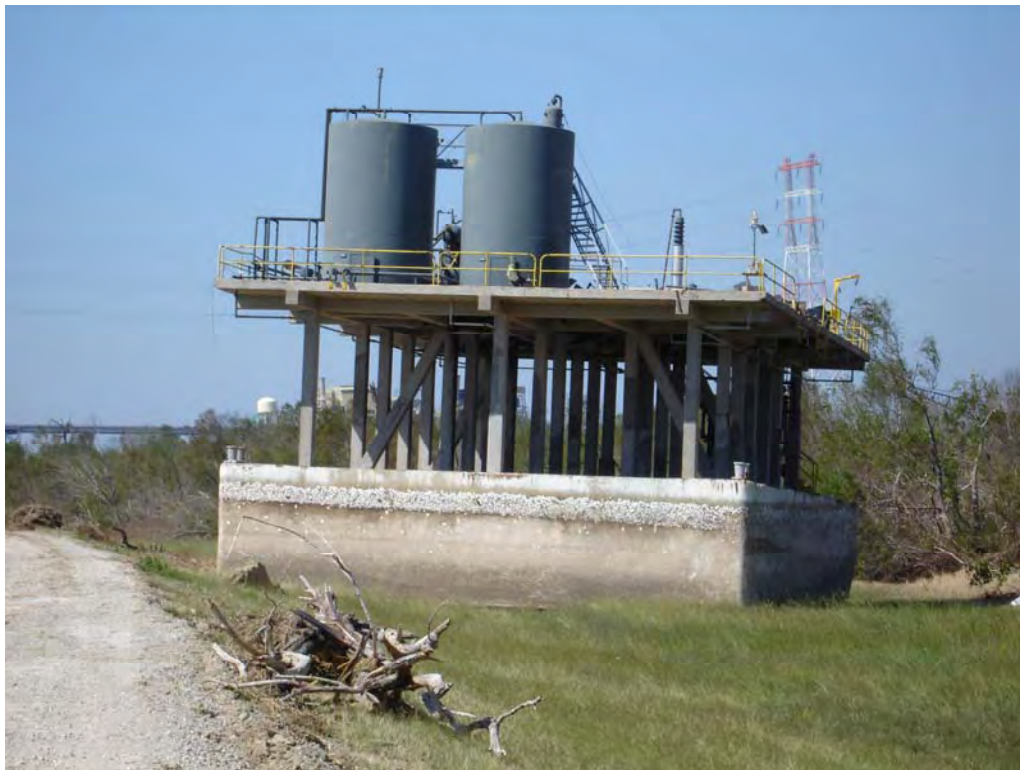
Fig. 18: Various barges and other floating structures made contact with the earth levees without causing significant damage. Photo shows a gas processing barge. (F. Silva, October 1, 2005).
