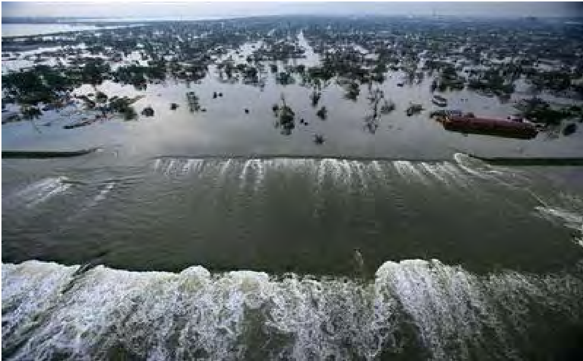
Figure 1.7: Flooding at the west end of the Ninth Ward, and outflow through levee breach as initial storm surge subsides.
