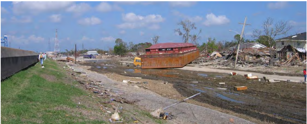
Fig. 4.5 - A barge was drawn through the south breach of the Lower Ninth Ward (J. Wartman, October 4, 2005).
