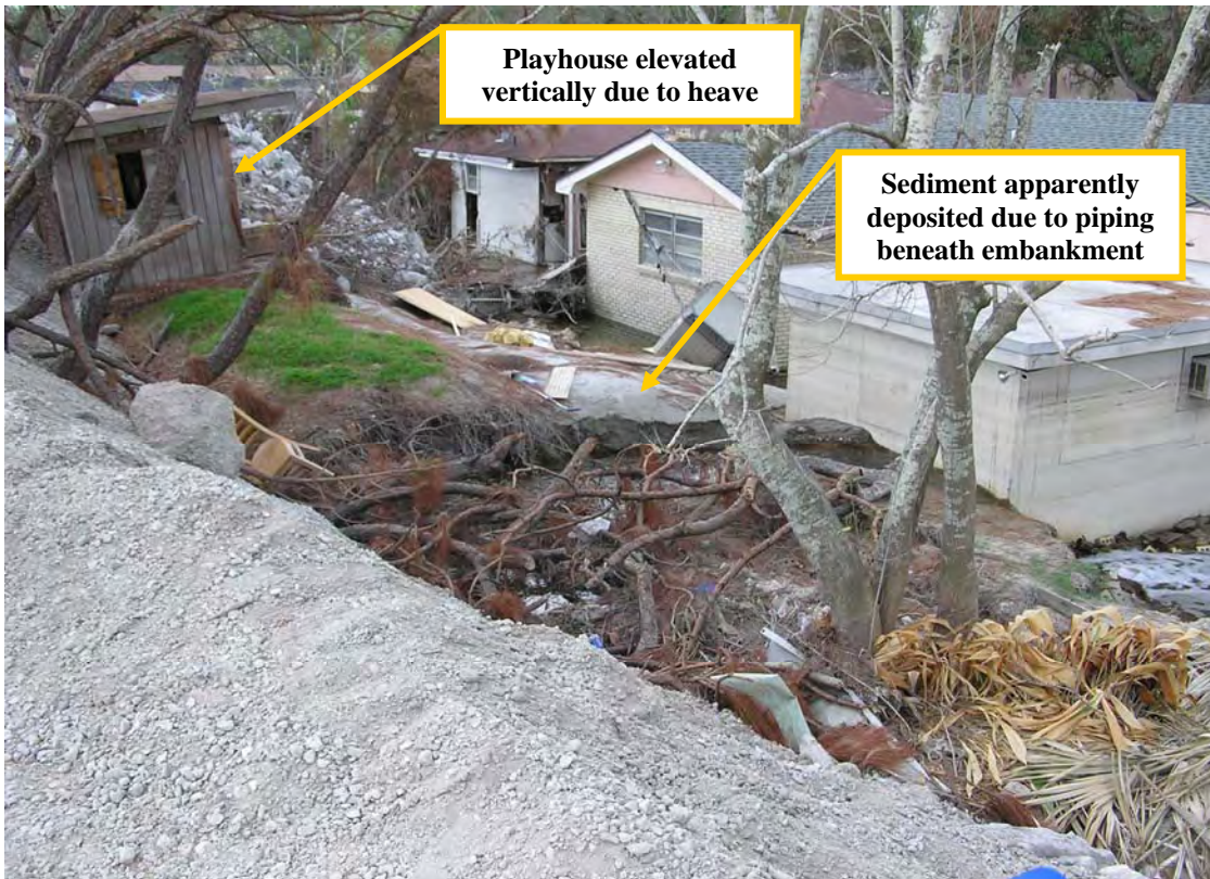
Figure 2.16: Conditions at the inboard toe of the London Avenue Canal (North) breach section.
