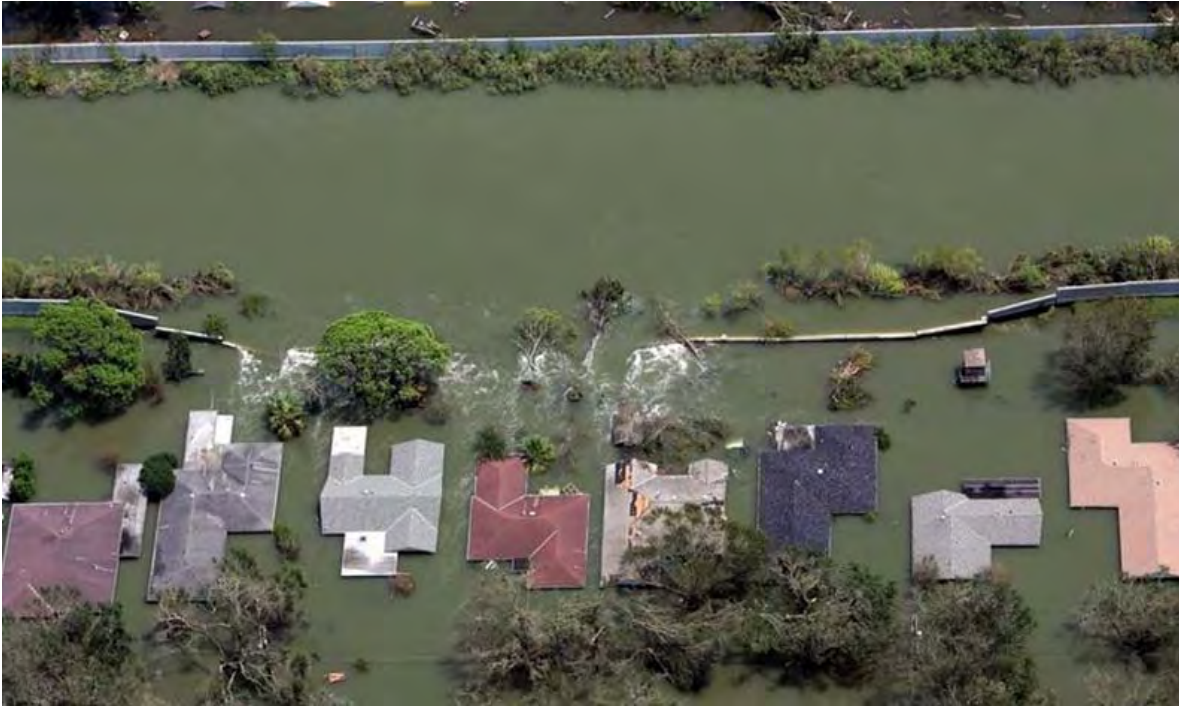
Figure 2.15: The breach section at the west side of the London Avenue Canal (North).
