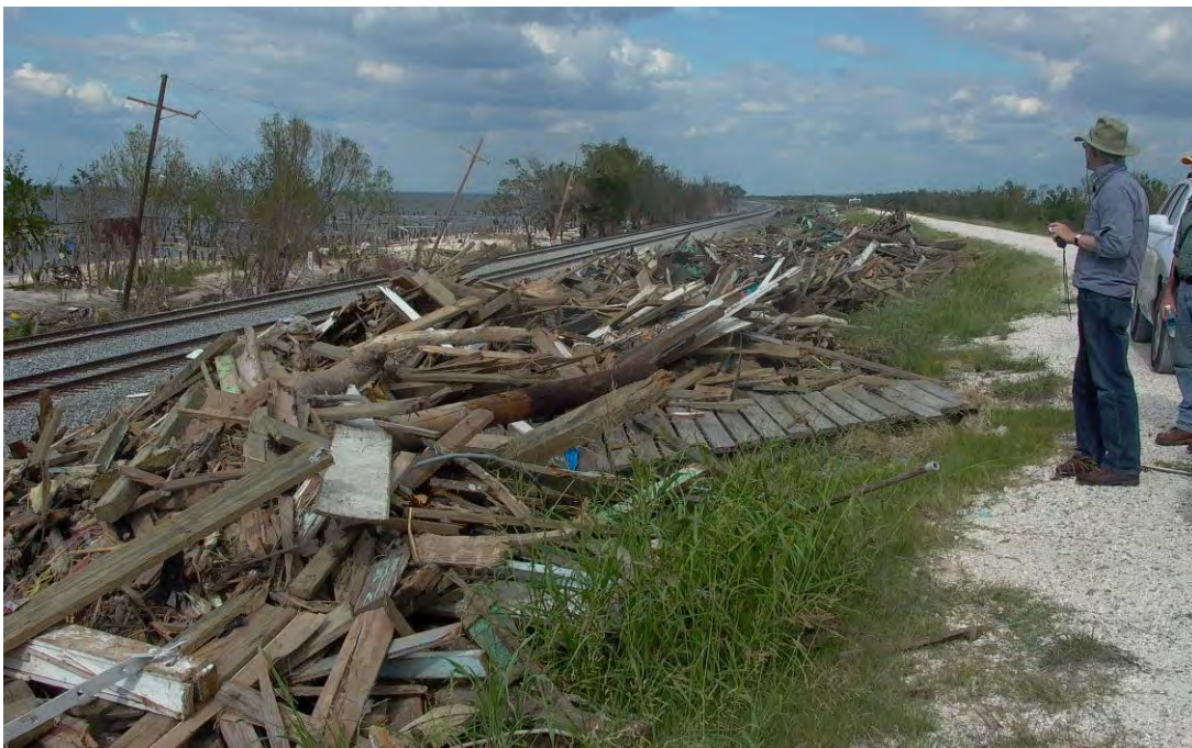
Figure 3.9: Debris from the Little Woods houses accumulated near the crest of the earth levee indicates the level of the lake waters during the storm. (Photo by F. Silva – N 30° 04' 70.5", W 89° 56' 44.0")
