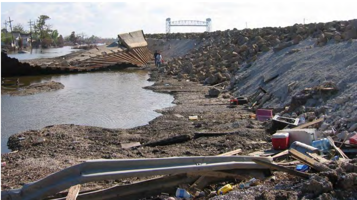
Fig. 4.11: Looking south of the north breach repair at the Lower Ninth Ward (J. Wartman, October 4, 2005).
