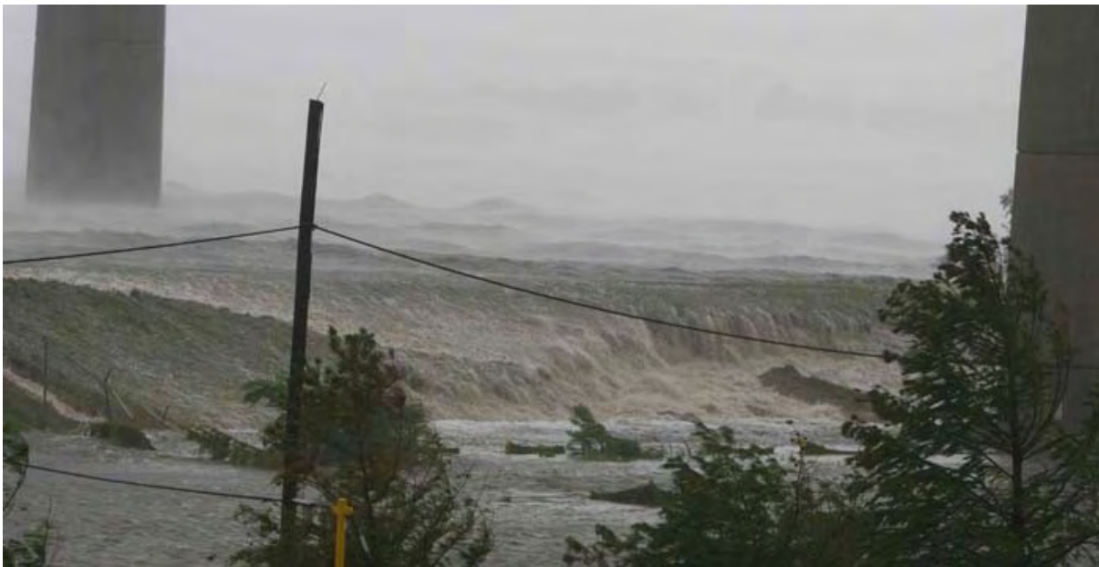
Photograph courtesy of Entergy Corporation
