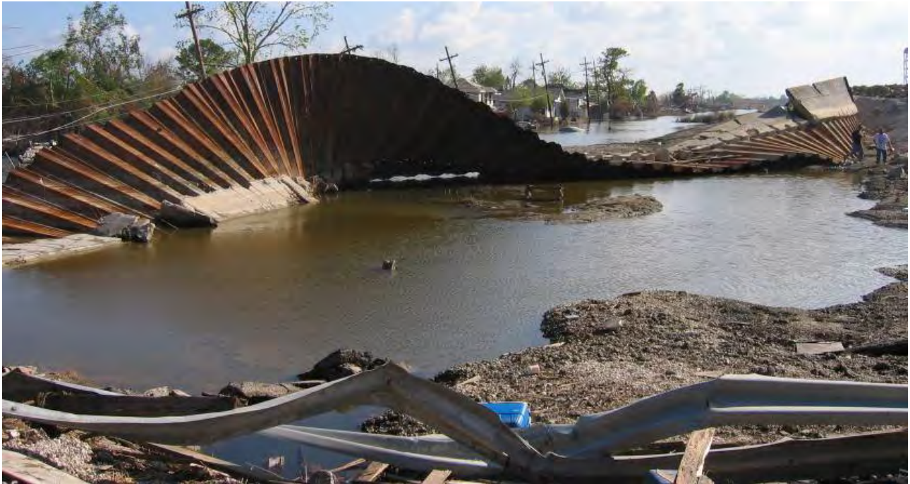
Fig. 4.10: Overturned I-wall system at north breach of Lower Ninth Ward (J. Wartman, October 4, 2005).
